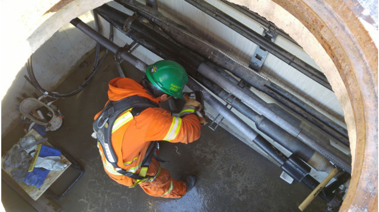
Figure 6.48 – Cable Splicing within a Cable Chamber
