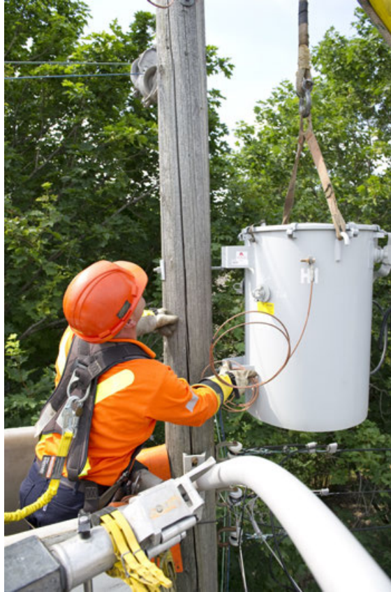
Figure 6.26 – Installation of Overhead Transformer
