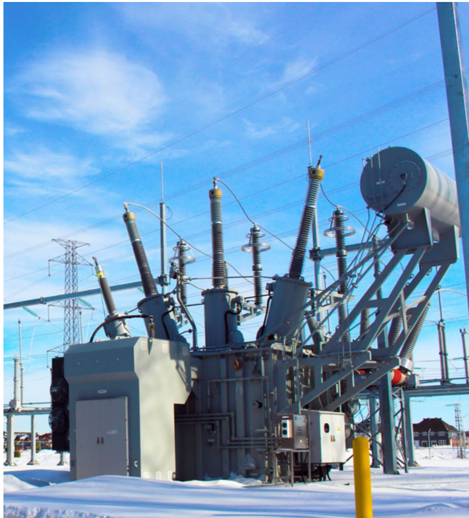
Figure 4.9 – Station Transformer at Terry Fox MTS
