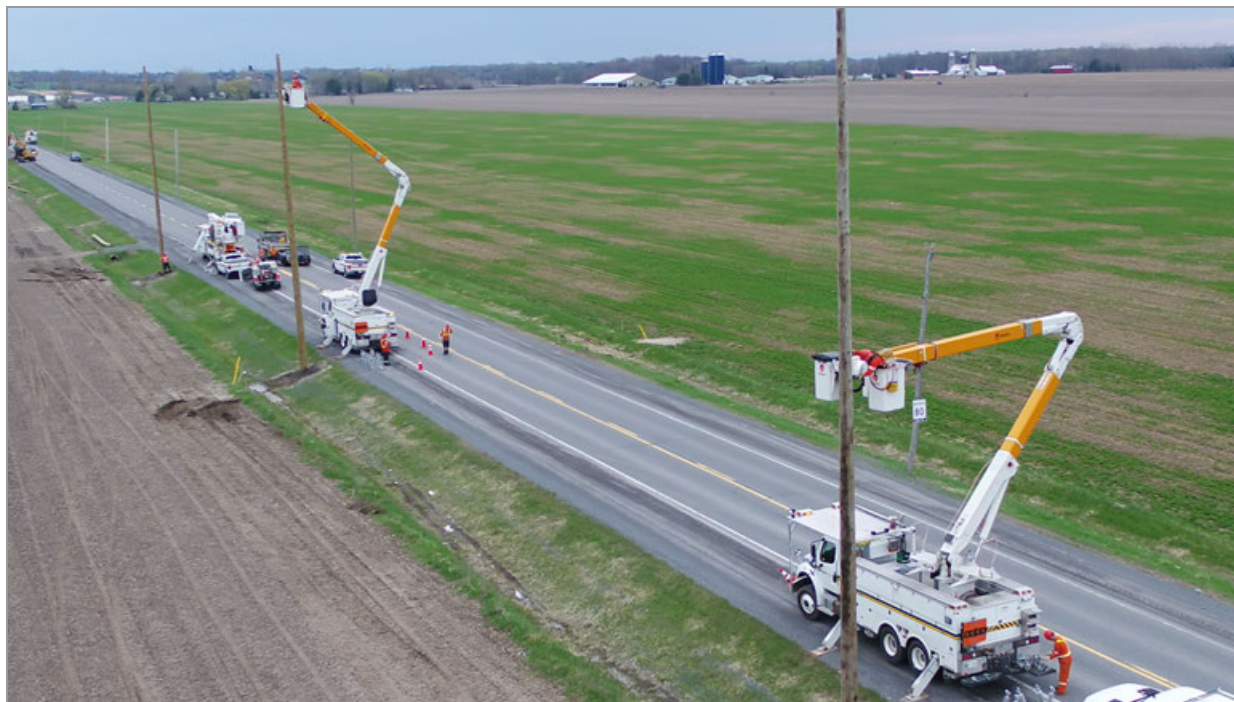
Figure 6.22 – Installation of New Pole Line
