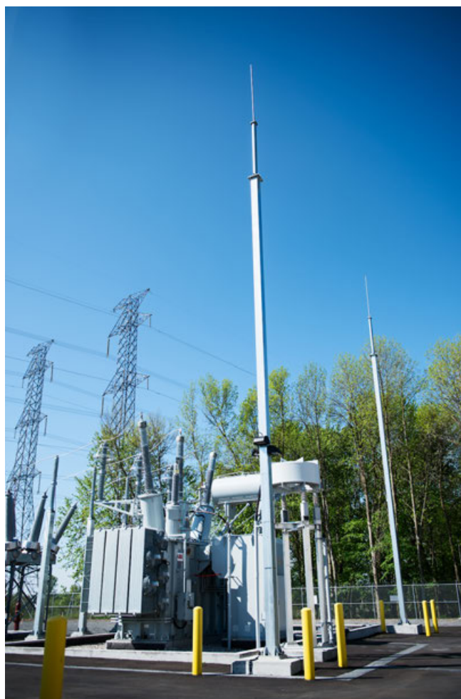
Figure 6.5 – 28 kV Station Transformer at Terry Fox MTS
