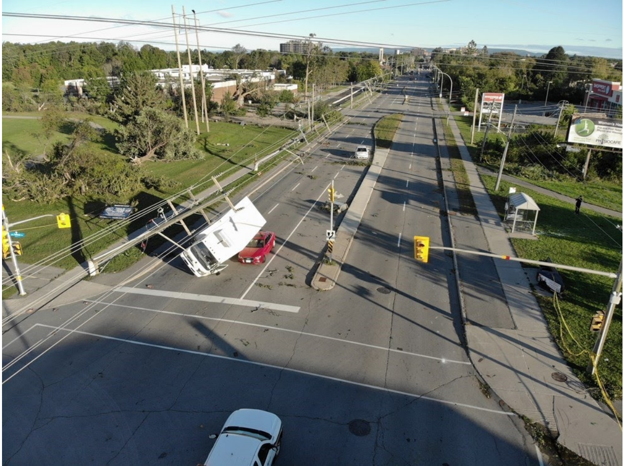
Figure 4.21 – Downed Pole Line Following September 2018 Tornado Event
