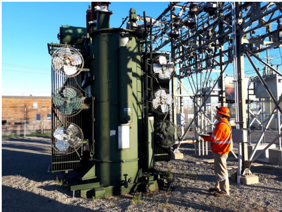
14 15 Figure 6.51 – Visual Inspection of a Station Transformer
