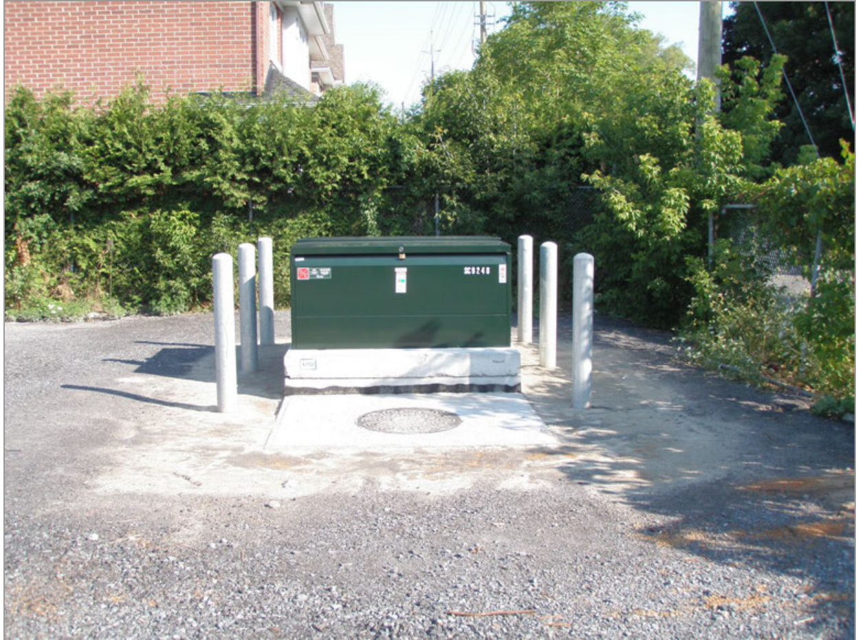
Figure 6.42 – Typical Installation of a Vista Type Underground Switchgear
