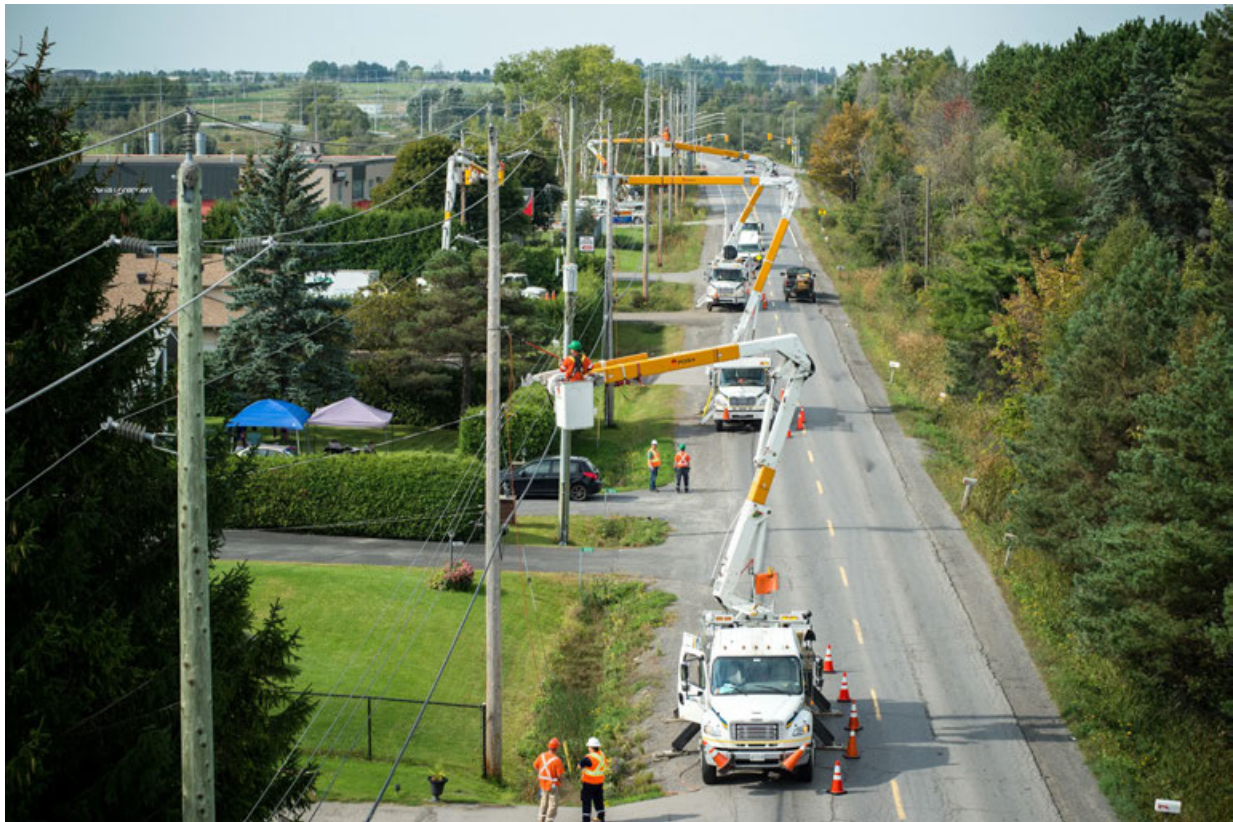
Figure 1.2 – Planned Insulator Replacement on 27.6 kV Pole Line
