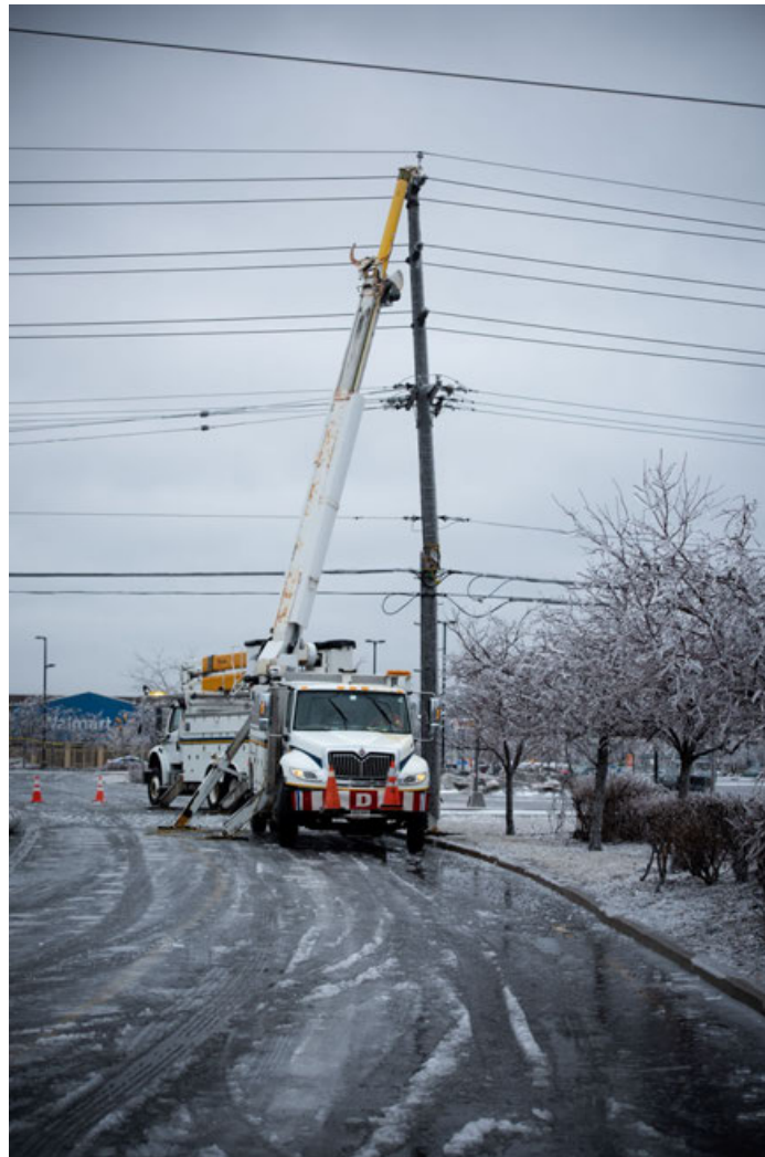
3 Figure 2.9 – Pole Replacement Following 2018 Ice Storm 4 5
