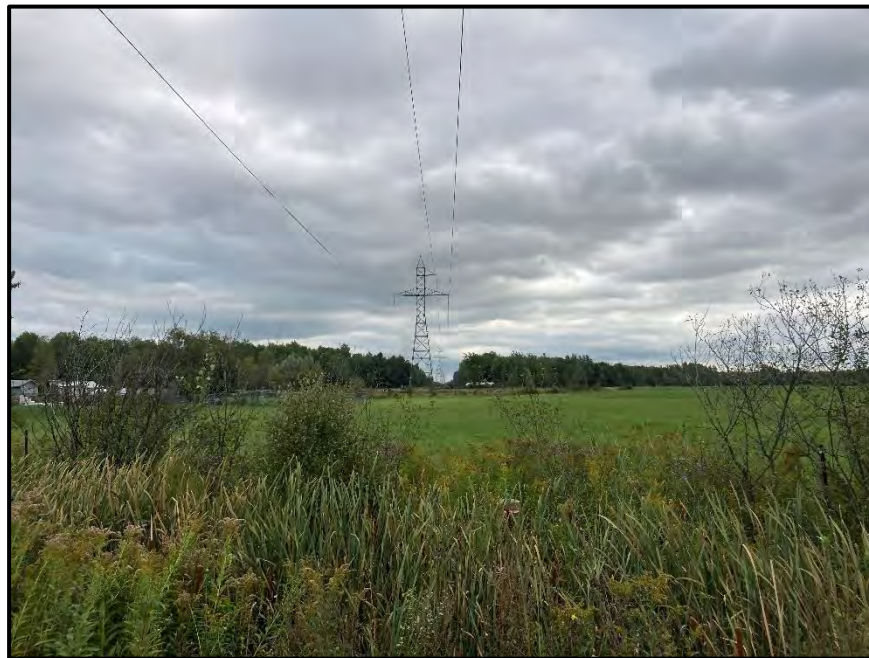
Image 8. View of a former farm field and saturated drainage ditch to the south of Thunder Road, looking southwest. (PR22-058D35)
