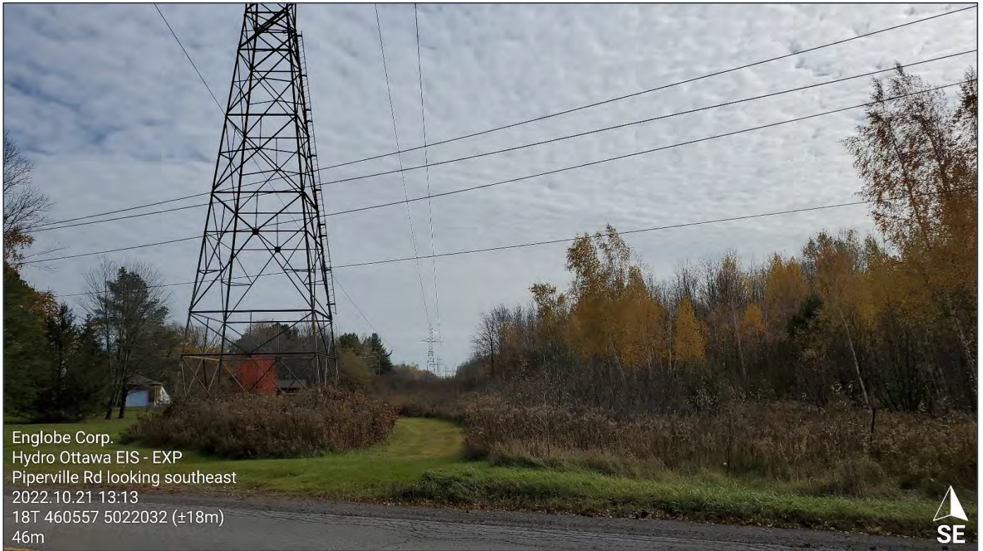
Site Photograph 5: Hydro One - L24A Corridor view looking south from Piperville Road.
