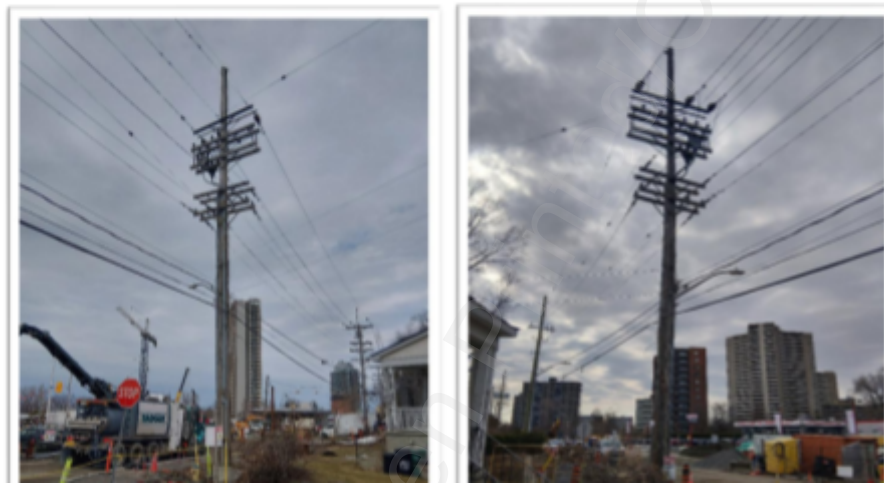
Figure 6-3. Example of Field Survey Notes & Photos
